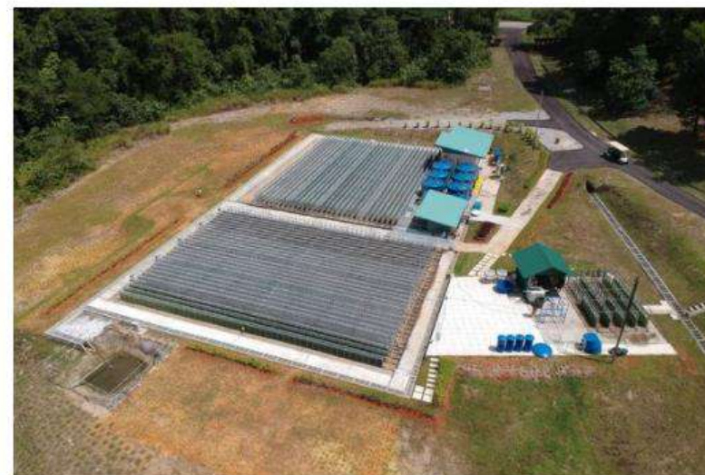
An algae cultivation facility in Malaysia. Source: Sarawak Biodiversity Centre
