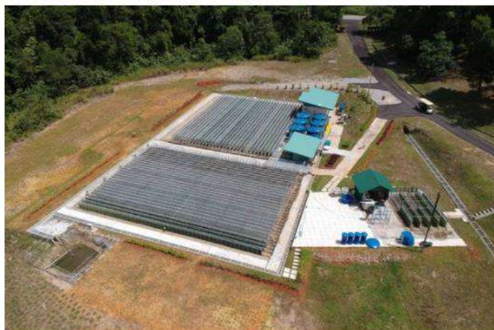
An algae growing facility designed by Chitose Group in Malaysia.
