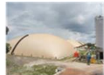
POME (Palm Oil Mill Effluent) Capture of biogas and Desulfurization Upgrading to bio-CNG by membrane treatment Handled as natural gas (CNG)
